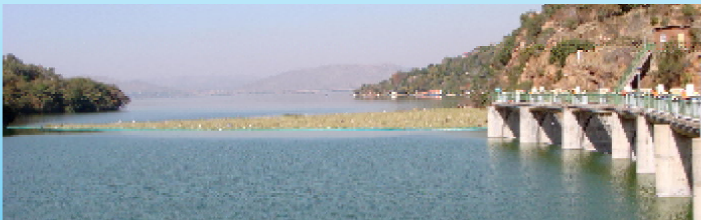
Prototype of boom at dam wall.
