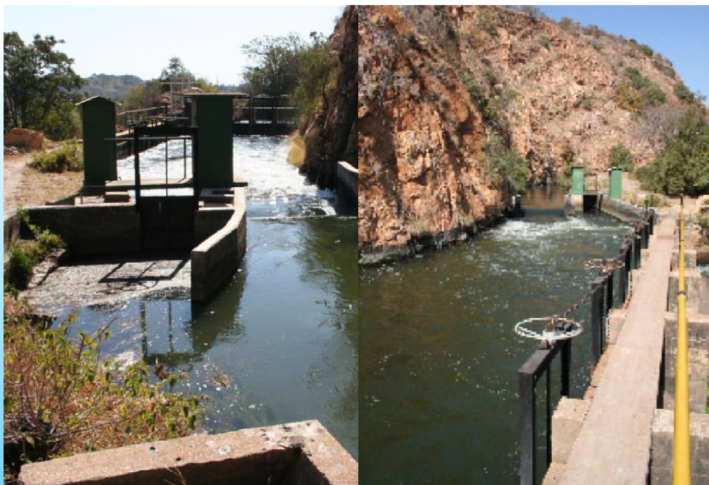
Water flowing from the dam into canals
